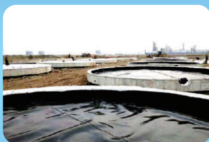
油罐罐底防渗 Oil Tank Bottom Anti-Seepage
